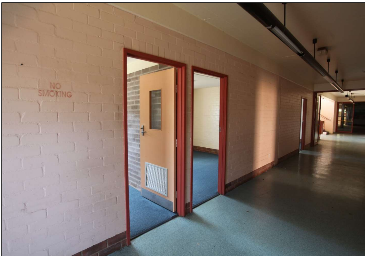
Figure 17: Typical internal design showing a mix of linoleum, carpet, timber doors, painted and face brick with plaster ceilings (Block A – Level 1)
