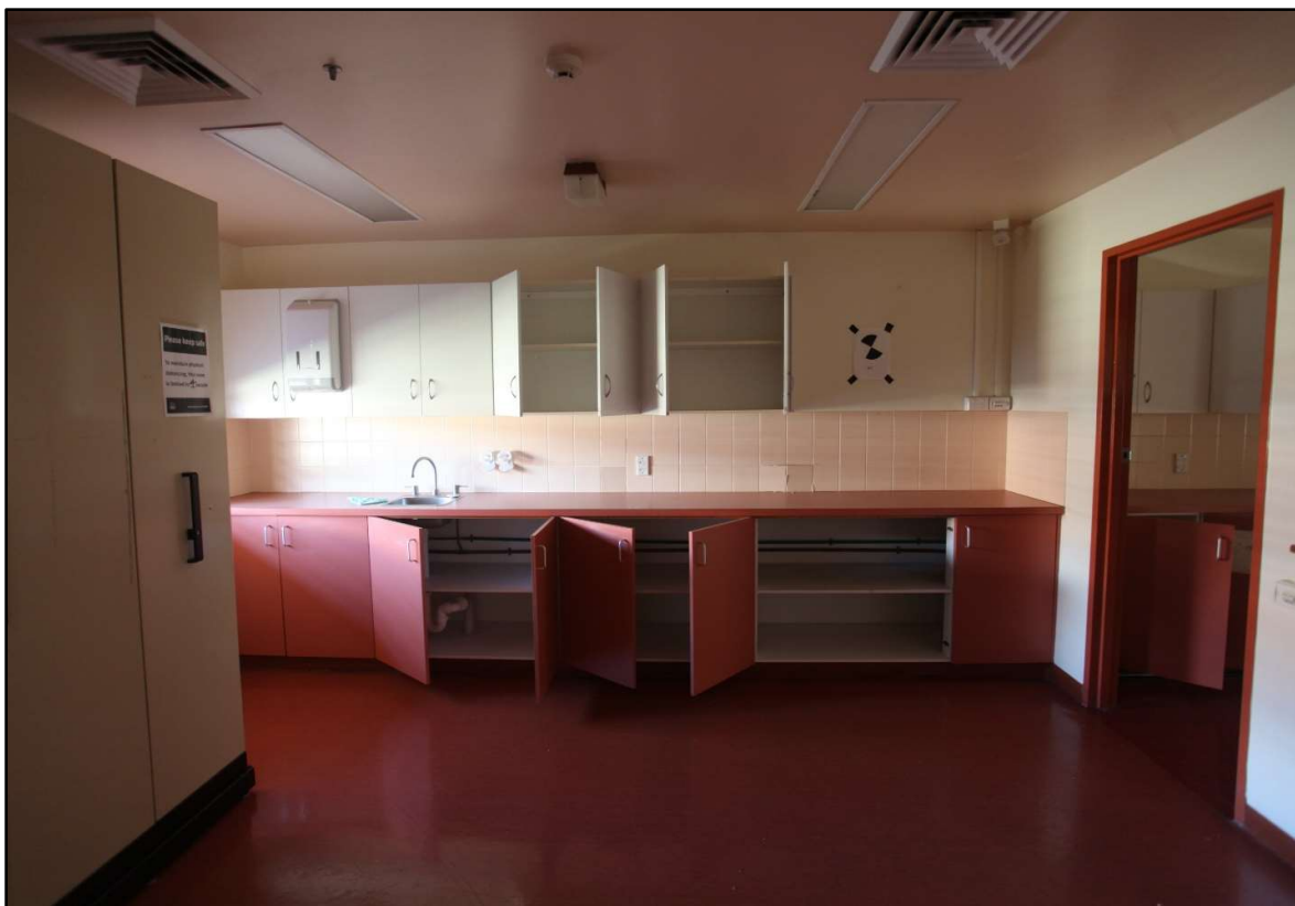
Figure 25: Kitchenette showing typical Laminex finish with tile splashbacks (Block B- Level 1)
