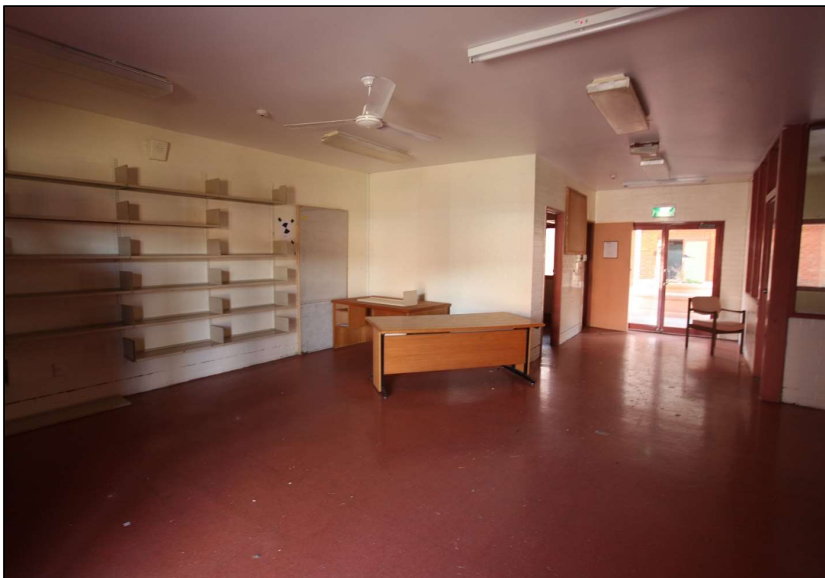
Figure 21: Typical internal fit out of painted brick, lino floor finish and plaster ceiling (Block B- Level 1)
